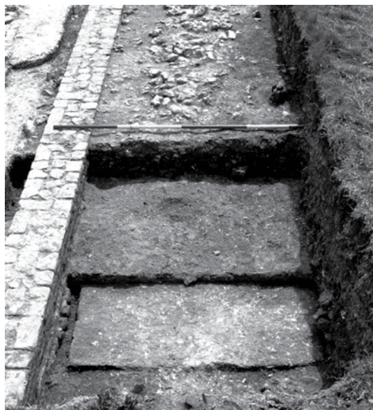
Fig. 12 Construction sequence: the wide footings trench ( 08 ) for lodge wall 07 is cut through grey clay subsoil ( 37 ). Mortar layer 34 and stones and soil 21 were deposited after the wall was built. Scale 2m
