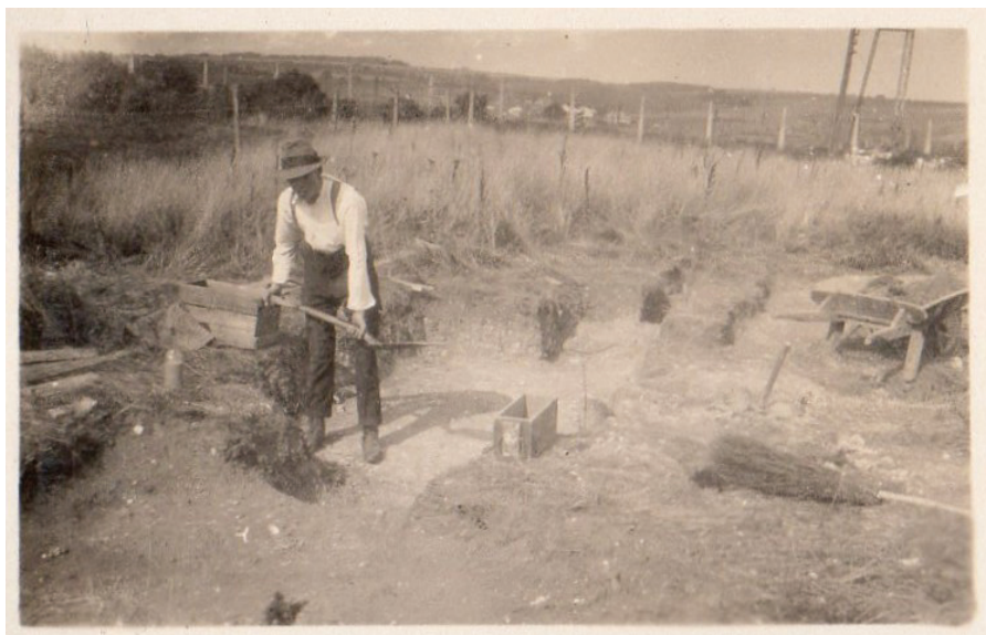
Fig. 1 R. C. Blake excavating at Woodham's Farm c 1925
