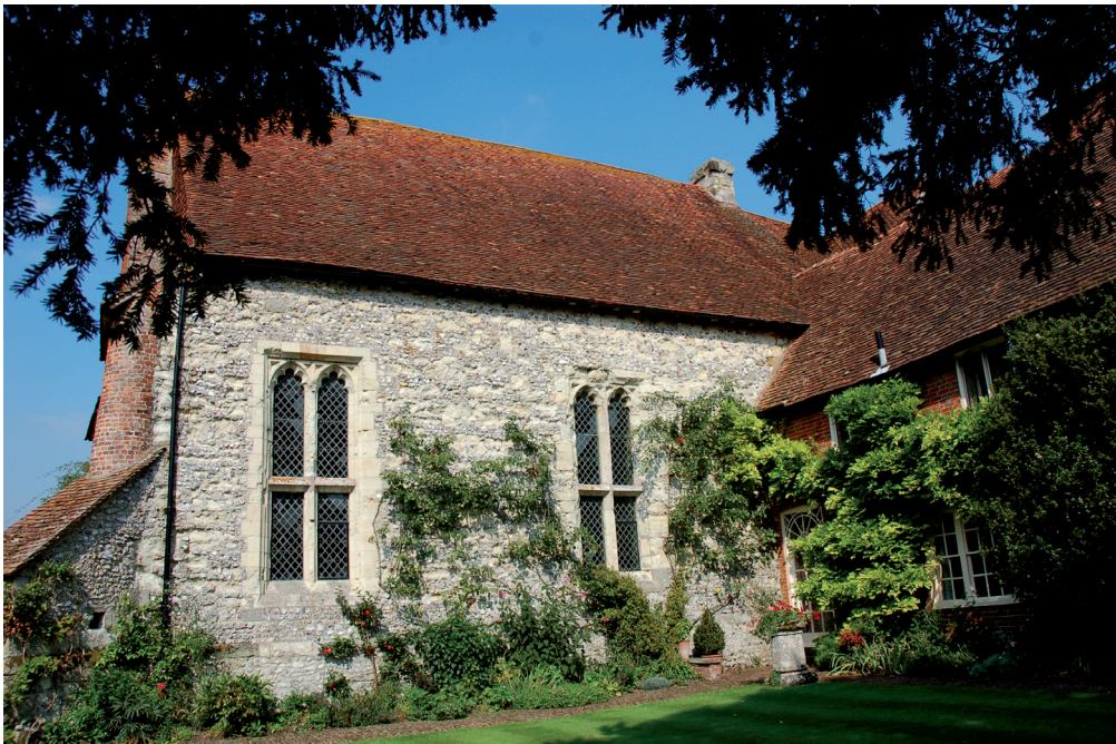
Fig. 3 Exterior of The Court Hall, built by Bishop William of Wykeham 1392 – 95. 'The best preserved of the Bishops' Palaces in Hampshire' (Pevsner)
