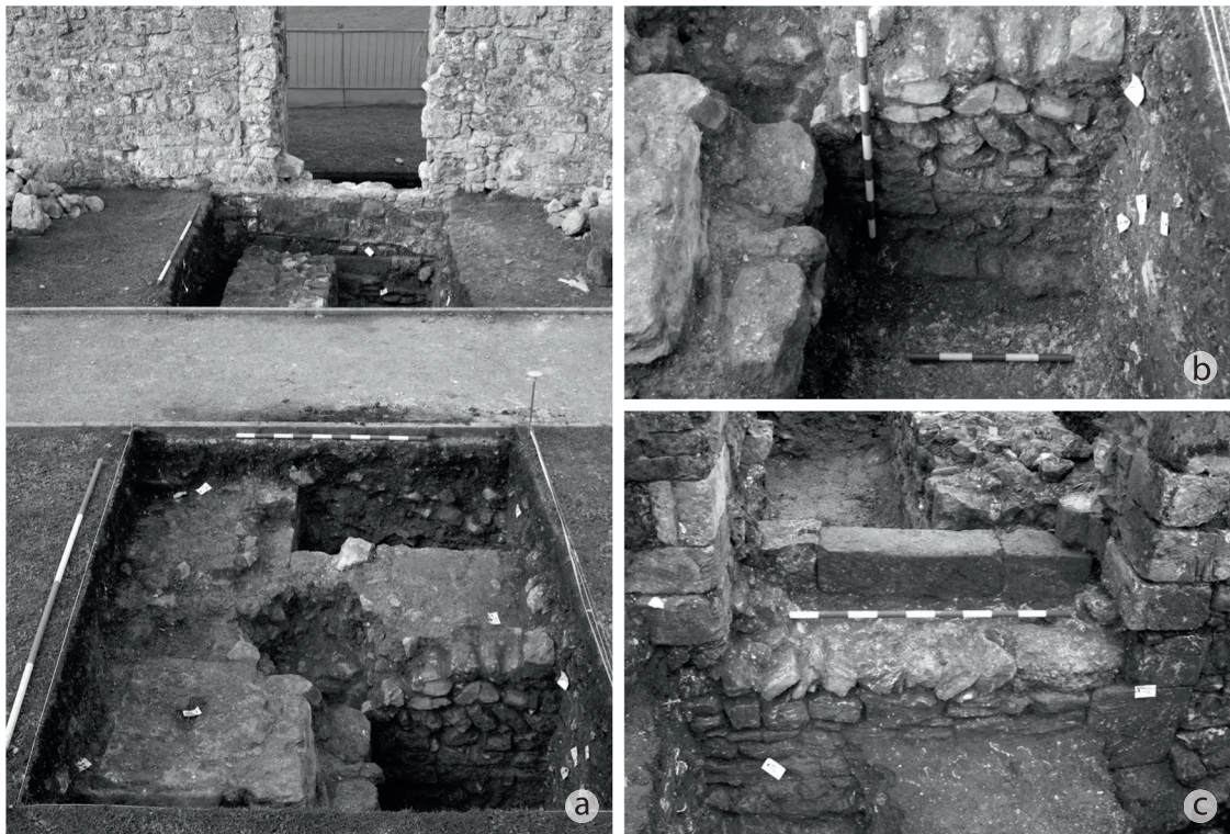
Fig. 13 (a) South gable end of Building 7347 and butress 7320 looking west. Note the straight joint in the 'garden' wall just left of the reopened entrance; (b) detail of Romanesque work in wall 7314 and the offset foundation of butress 7320 which it butts; (c) detail of Romanesque work and staggered quoins in wall 7346 showing the sill of the 19th century gateway
