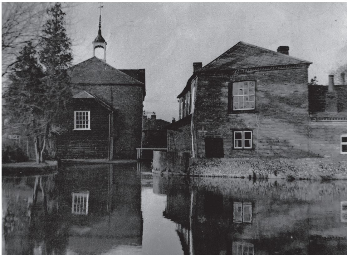
Fig. 10 The two-storey building and the cottages from the south. The south-west corner was later reinforced with a buttress because of subsidence. The straight joint between the building and the cottages shows that they post-dated it
