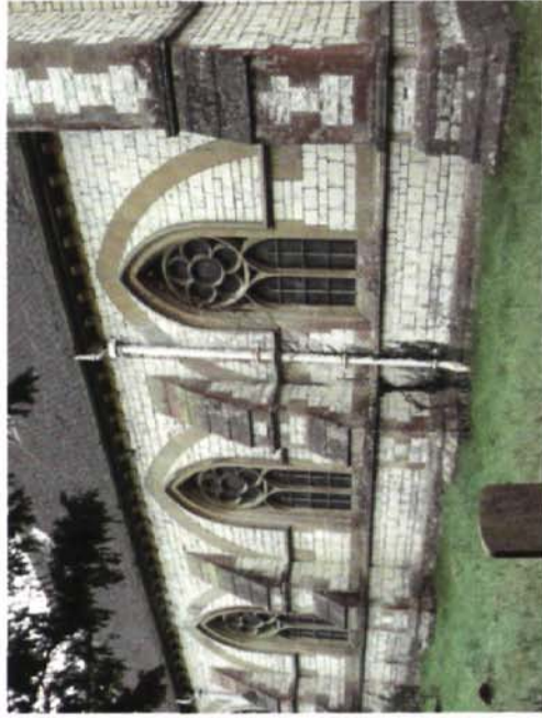
Fig 10 Chalkland churches. A – St. John the Baptist (1875), Greatham, faced in randomly arranged blocks of chalk with Bathstone dressings, from the southeast. B – Facing of random blocks of chalk, All Saints (1876), Kingsley. C – Facing of neatly coursed and varied, dressed chalk, St. Matthew (1868), Blackmoor. D – St. James, (1839), Bossington, flint with mainly Caenstone dressings, from the southeast. Note the roofing of graded stone slabs
