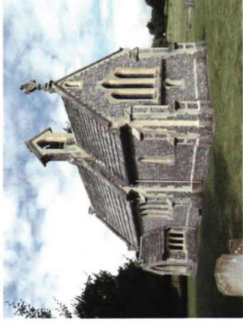
Fig 10 Chalkland churches. A – St. John the Baptist (1875), Greatham, faced in randomly arranged blocks of chalk with Bathstone dressings, from the southeast. B – Facing of random blocks of chalk, All Saints (1876), Kingsley. C – Facing of neatly coursed and varied, dressed chalk, St. Matthew (1868), Blackmoor. D – St. James, (1839), Bossington, flint with mainly Caenstone dressings, from the southeast. Note the roofing of graded stone slabs
