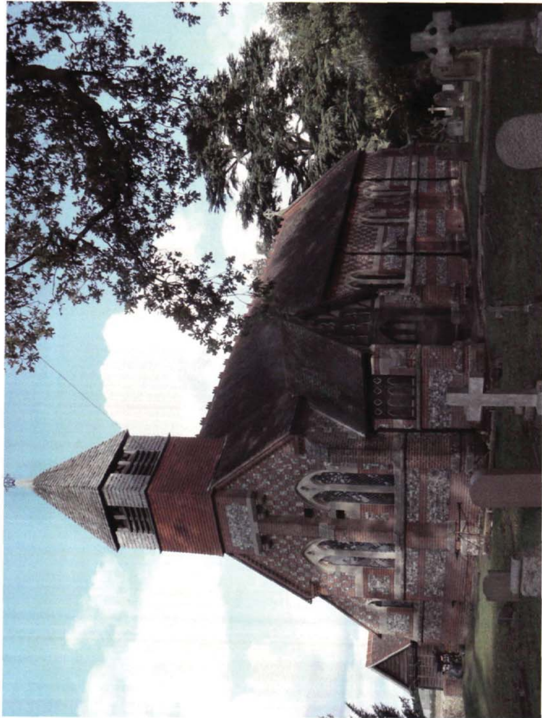
Fig 14 St. Mary (1867), Beech Hill, flint with a variety of decorative brick in chequers and bands
