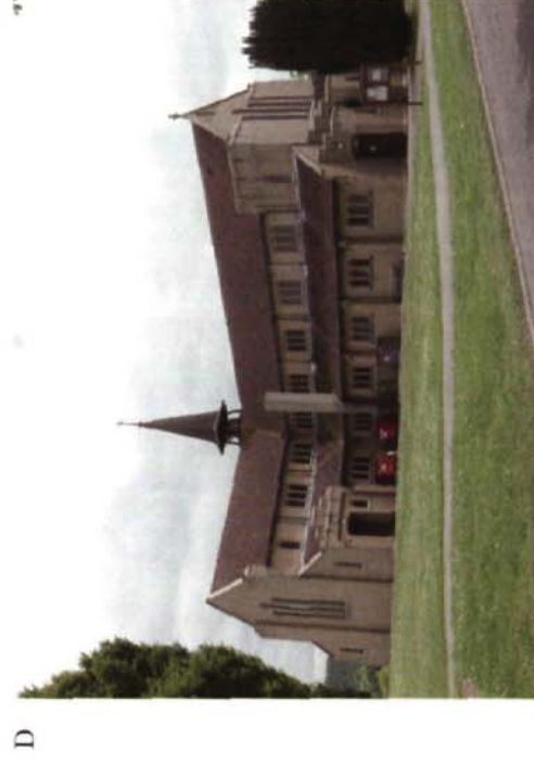
Fig 16 Chalkland churches. A – St. Mary (1768–71), Avington, red brick with Portland limestone dressings, from the southeast. B – St. Michael (1775), Crux Easton, blue and red brick, from the southwest. C – All Saints (1863), Aldershot, red brick with Bathstone dressings, from the southeast. D – St. Michael (1912), South Tidworth, faced wholly in terracotta, from the southwest
