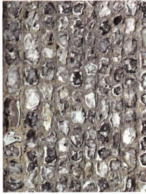
Fig 13 Varieties of flint facings in chalkland churches. A – Coursed, dressed flint, St. Peter (1845), Brown Candover. B – Shingled, flint nodules, St. Lawrence (1864), Wootton St. Lawrence. C – Roughly coursed, broken and split flint nodules, St. Mary (1866), Lasham. D – Roughly coursed, mainly broken flint nodules, St. Michael (1869–70), Highclere
