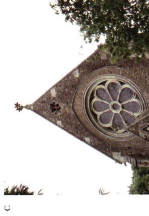
Fig 9 Chalkland churches. The gabled chancel (A), nave (B) and west window (C) of St. Mary (1861), Ichen Stoke, in Bargate stone with Bathstone dressings
