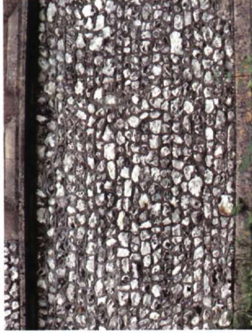
Fig 13 Varieties of flint facings in chalkland churches. A – Coursed, dressed flint, St. Peter (1845), Brown Candover. B – Shingled, flint nodules, St. Lawrence (1864), Wootton St. Lawrence. C – Roughly coursed, broken and split flint nodules, St. Mary (1866), Lasham. D – Roughly coursed, mainly broken flint nodules, St. Michael (1869–70), Highclere
