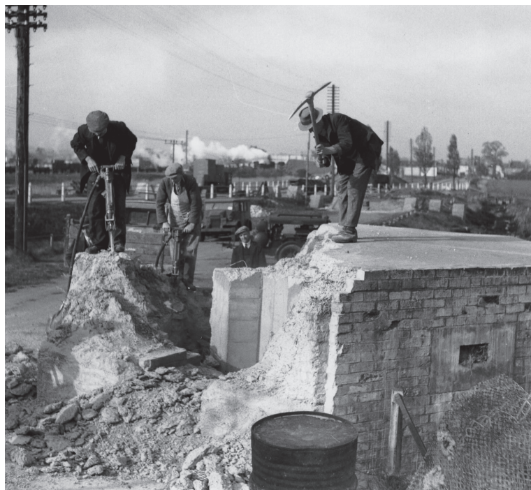
Fig. 6 Pill-box demolition to widen the Southampton – Hythe road (30/4/1944) (IWM H 38318)
