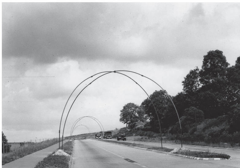
Fig. 3 Aerial obstructions across carriageway (June 1940) (IWM H 2067)
