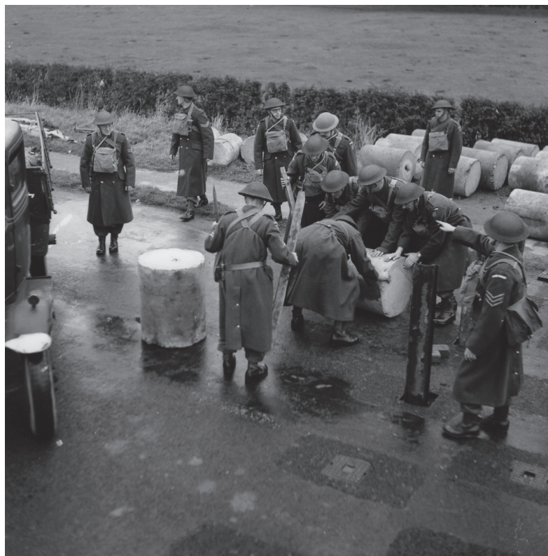
Fig. 2 Home Guard placing concrete anti-tank cylinders – note metal sockets in carriage way into which metal rails are being inserted (IWM H 15192)
