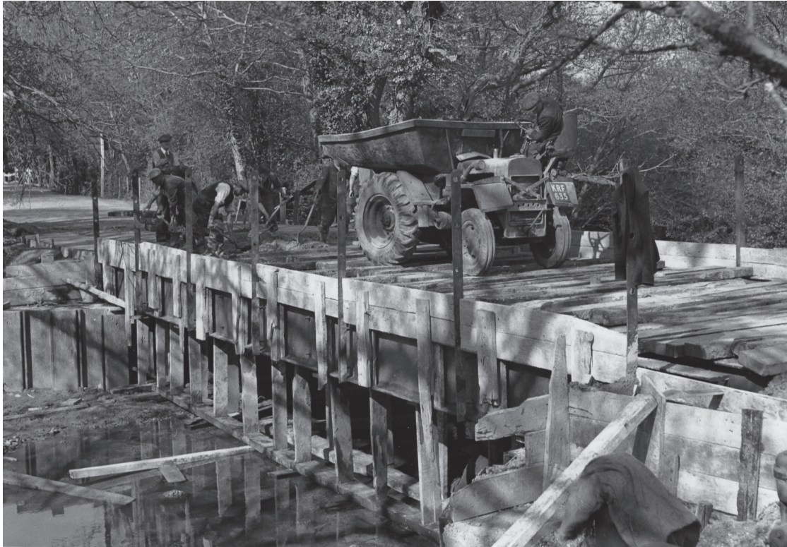
Fig. 8 Replacement reinforced concrete bridge on Brockenhurst – Beaulieu road (1/5/1944) (IWM H 38320)
