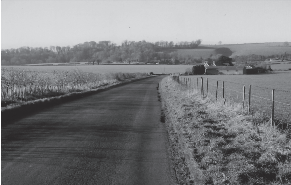
Fig. 9 Brook Lane (C 200), Hambledon – widened for troop movements to and from camp at Grenville Copse. Now used for motorists travelling between Clanfield and the A32 (Photograph, M Walford)
