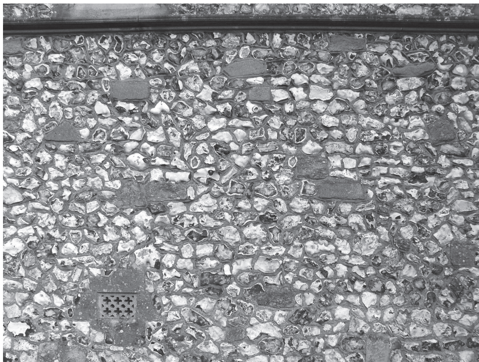
Fig. 2 Partly dressed blocks of Ham Hill stone in the flint facing at St. Mary's Laverstoke
