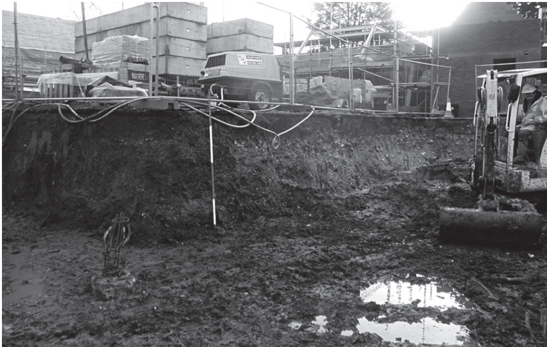
Fig. 11 ( below ) New swimming pool showing rubble filling of possible medieval fishpond
