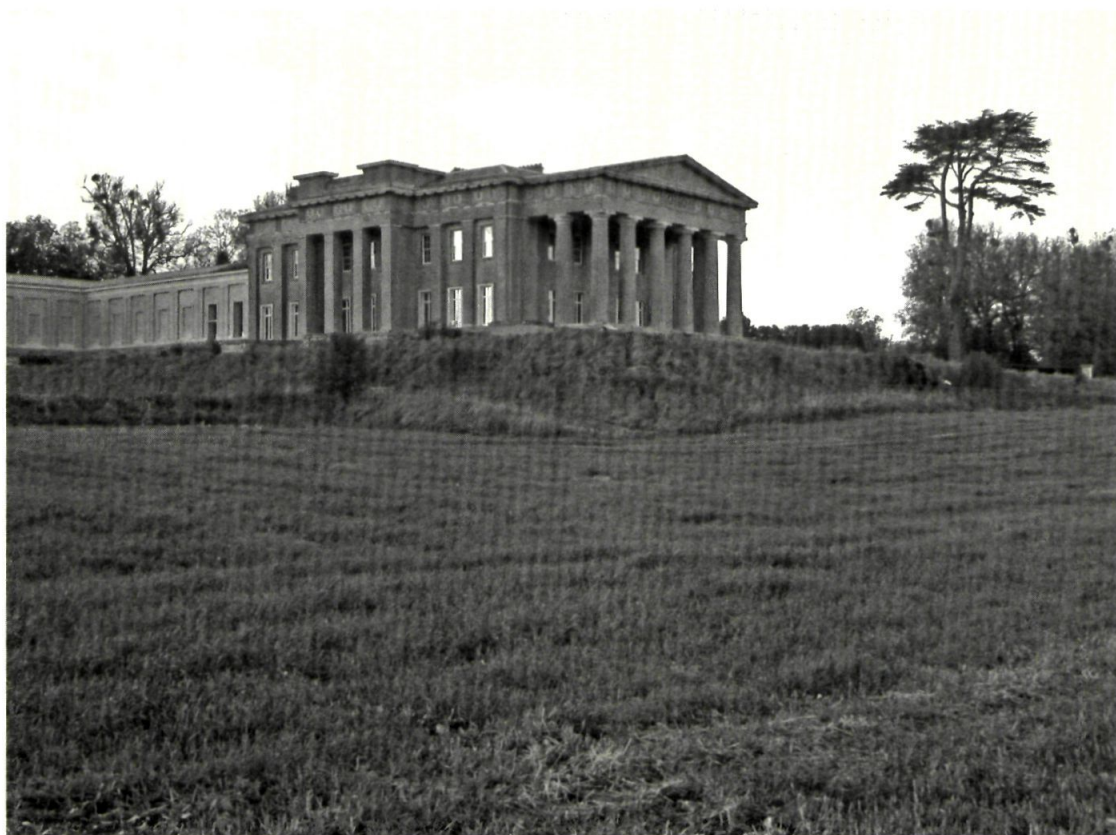
Fig. 2 Linear features underlie the foreground of this view of The Grange
