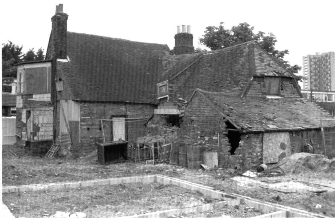
Fig. 4 Ivy House prior to restoration seen from the rear. The timber-framed structure is contained within the projecting wing to the right.
