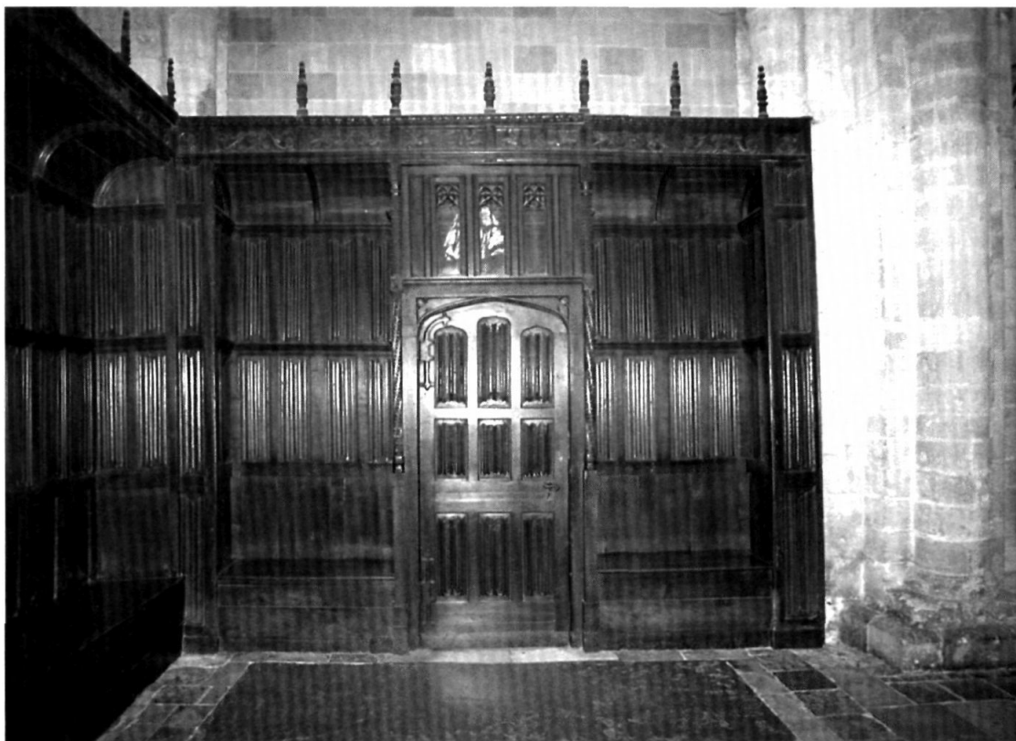
Fig. 1 West side of the south transept showing Silkstede's frieze above three tiers of panelling with early nineteenth-century door and frame.
