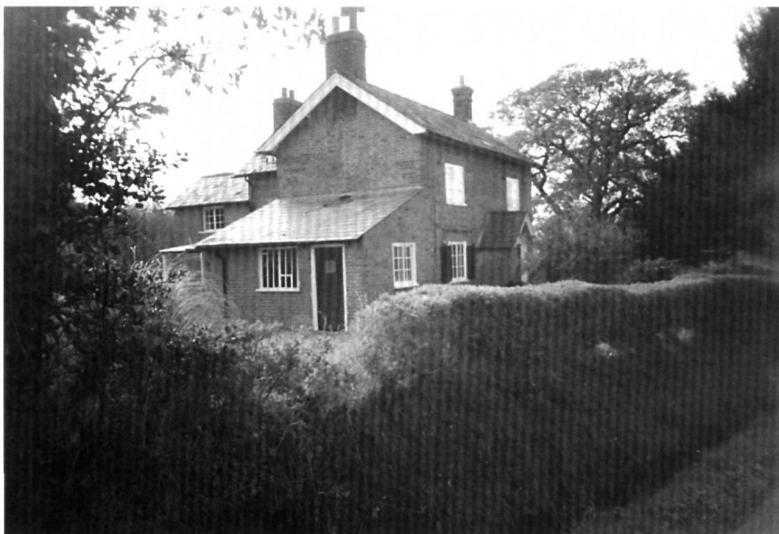
Fig. 4 Cottage at Middle Toothill, the brickwork showing evidence of an upper floor having been added. (Photo R Hayden)
