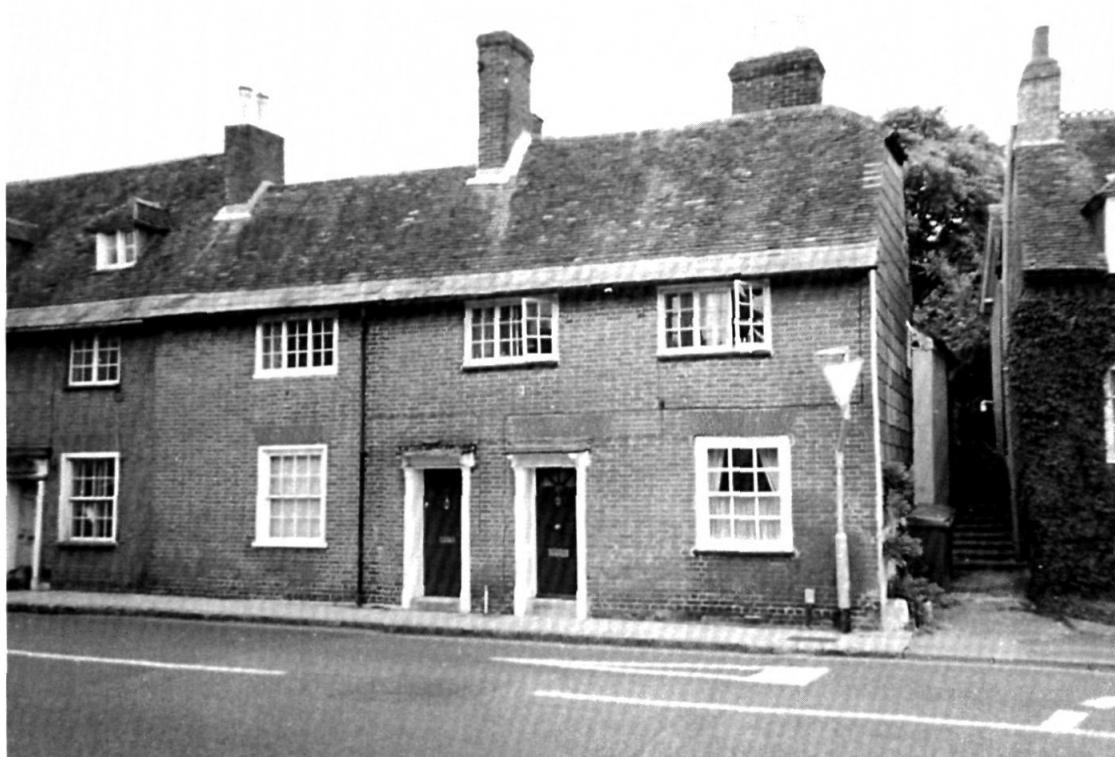
Fig. 3 Nos 26 and 28 Palmerston Street: original window placement on ground floor indicated by gauged brickwork, with later insertion of a door. Upper storey shows movement of windows on right side as now out of line with gauged brickwork below. (Photo R Hayden)
