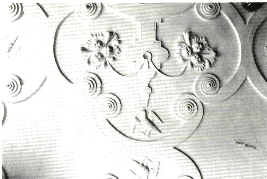
Fig. 5 Detail of plaster ceiling showing ribs and repetitive ornament
