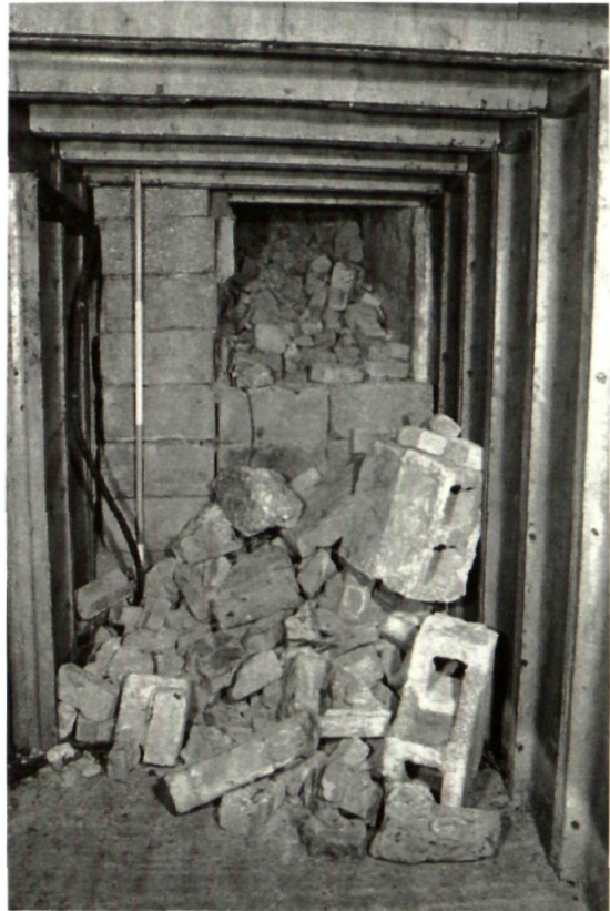
Fig. 7 Blocked entrance in the southern shelter, Jewry Street, Winchester (Context One Archaeological Services 1998)
