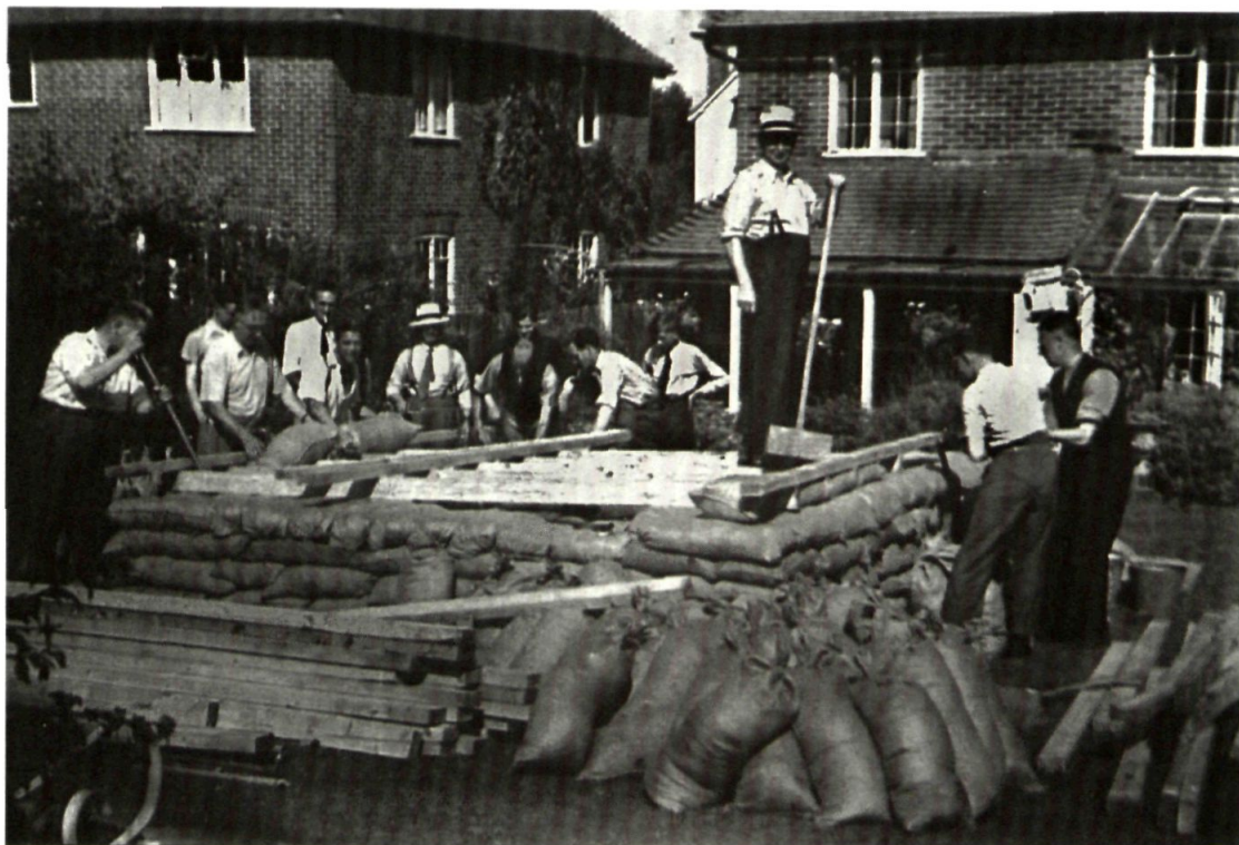
Fig. 1 Work on an ARP Warden's shelter at the junction of Weston Road and Fordington Avenue (by kind permission of Mrs Sherriff)
