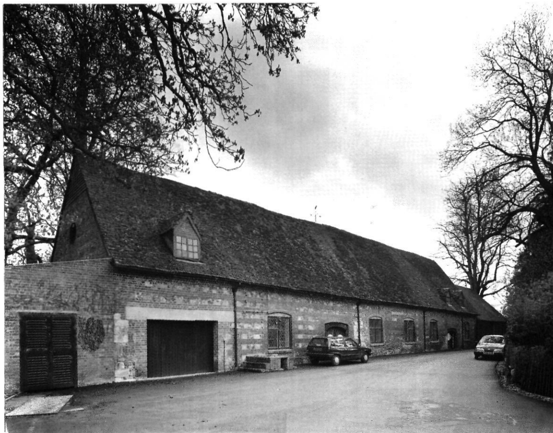
Fig. 4 Wherwell Abbey: 'The Stables' viewed from the north-east. The large limestone quoins to the left of the garage entrance could mark the original end of the 13th-century structure. Note the lower roof to the right which may have been to full height before a post-medieval rebuilding. (Photograph – John Crook)
