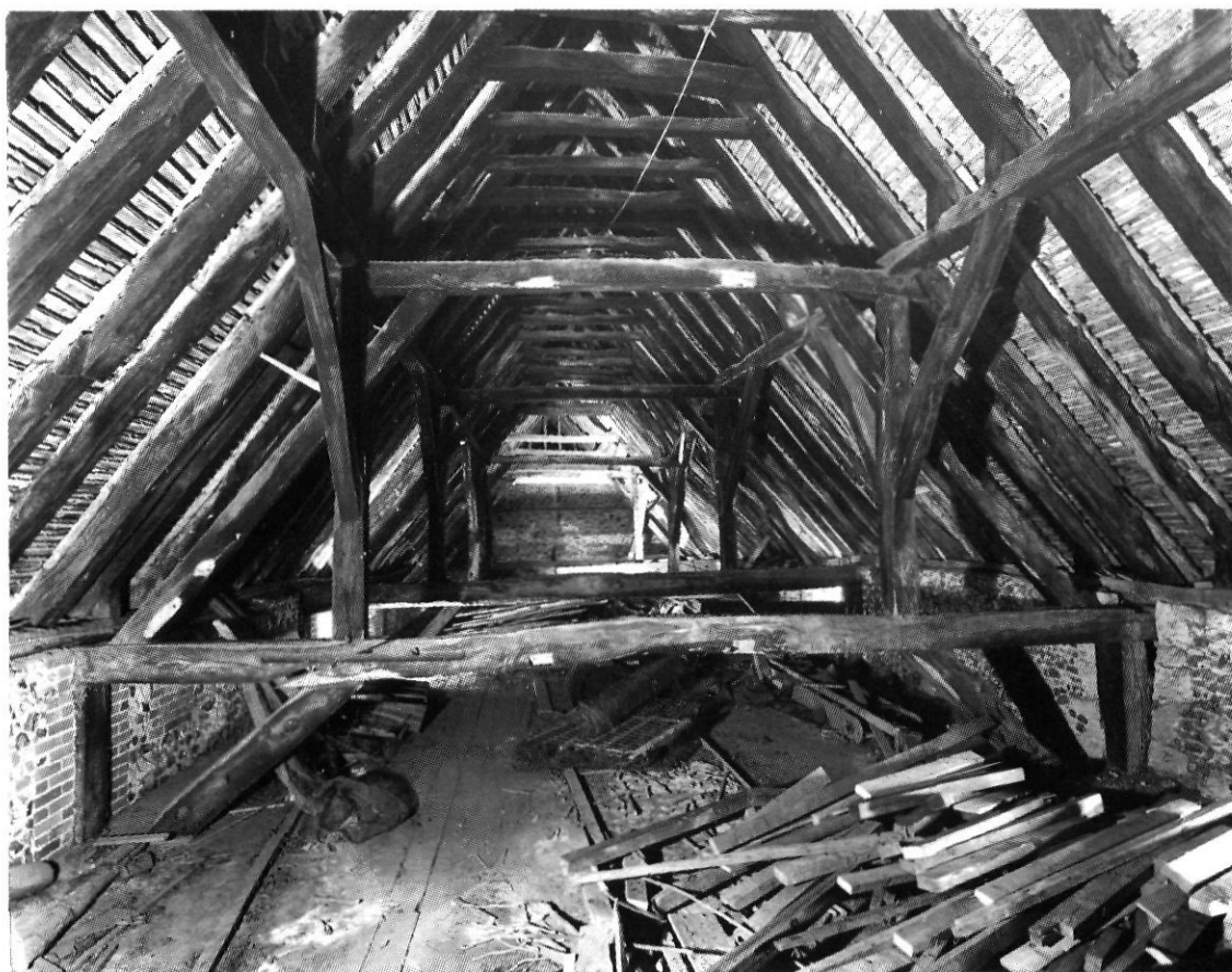
Fig. 5 Wherwell Abbey: the roof of 'The Stables' viewed from the west. In the foreground is truss 7 of the first building phase of 1250 – note the original scarf joint in the lower tie beam which has been reinforced with an iron strap. The three trusses of the second phase can be seen behind it. (Photograph – John Crook)
