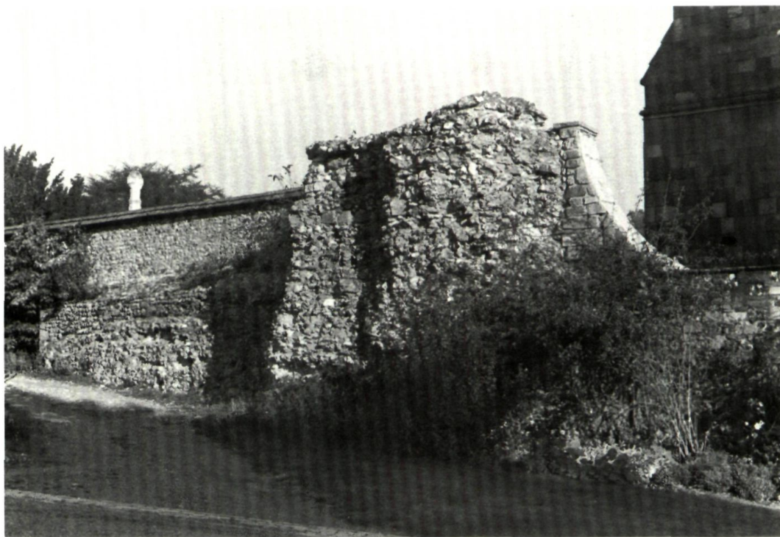
Fig 3. Winchester Cathedral. No 11, The Close, north face of north wall (photo: author)
