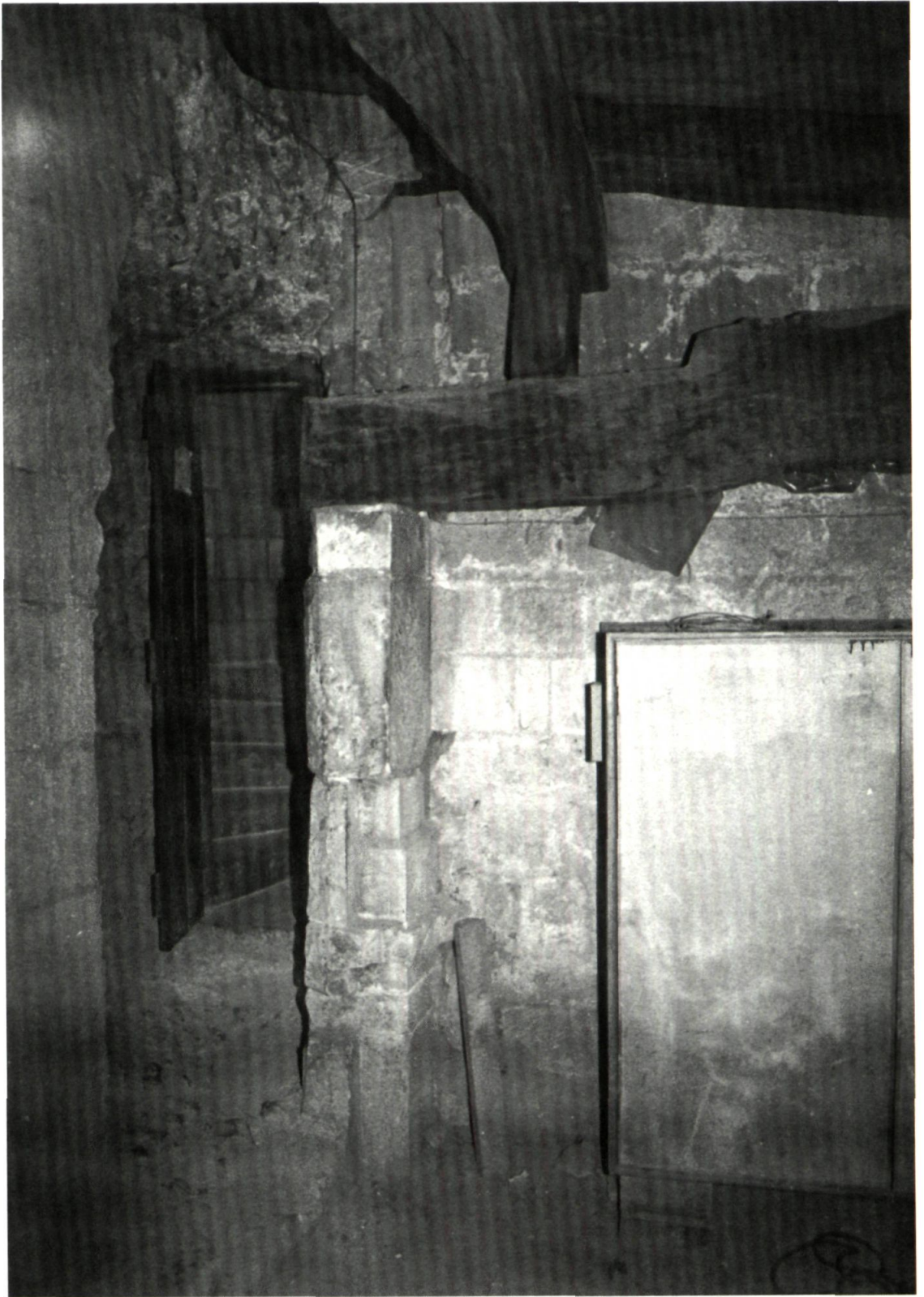
Fig 13. Winchester Cathedral. Entrance to north aisle roof space from fourteenth-century stair vice made in fifteenth-century through twelfth-century masonry (photo: author)
