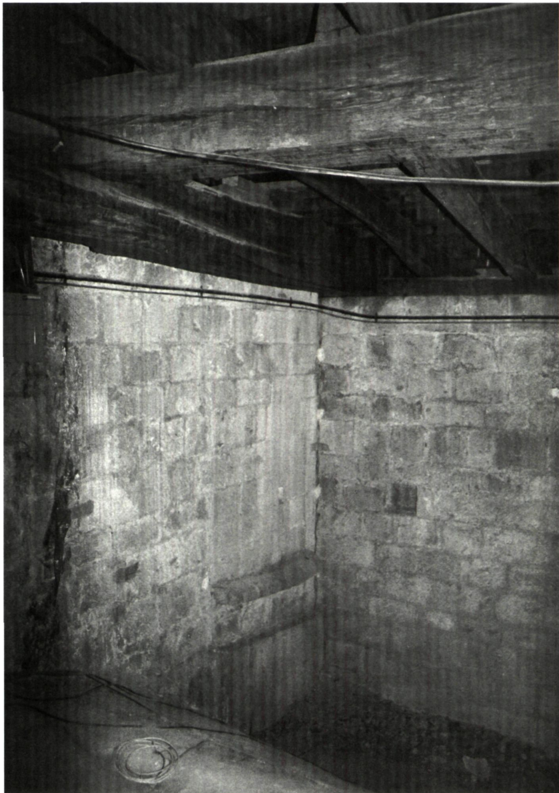
Fig 14. Winchester Cathedral. Junction of fifteenth-century north aisle wall with fourteenth-century west wall (photo: author)
