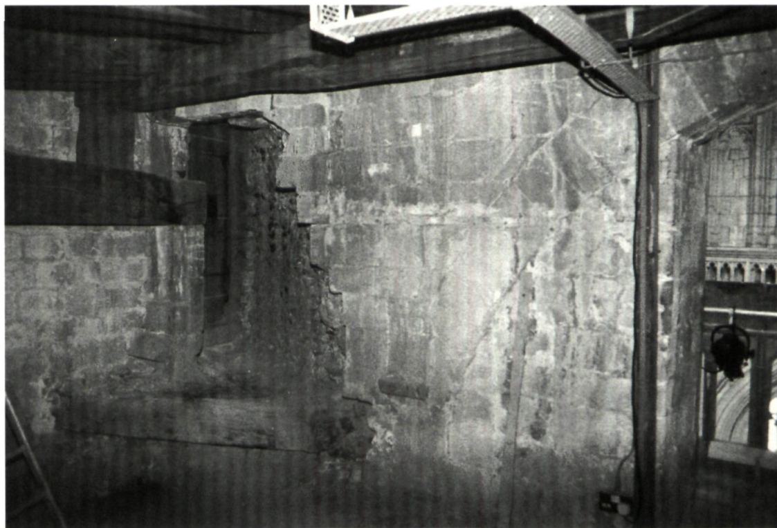
Fig 11. Winchester Cathedral. Remains of Romanesque gallery at west end, above south aisle vaults (photo: author)
