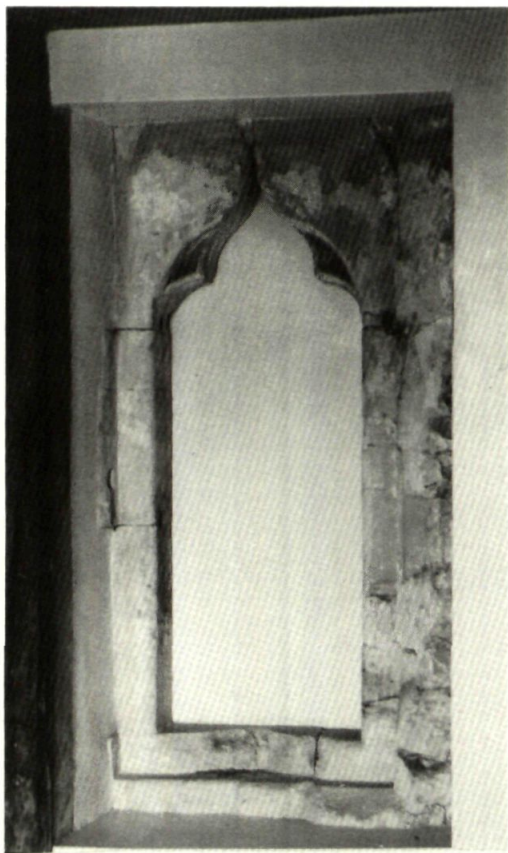
Plate 3. The refined Decorated window in the north wall of the solar range.
