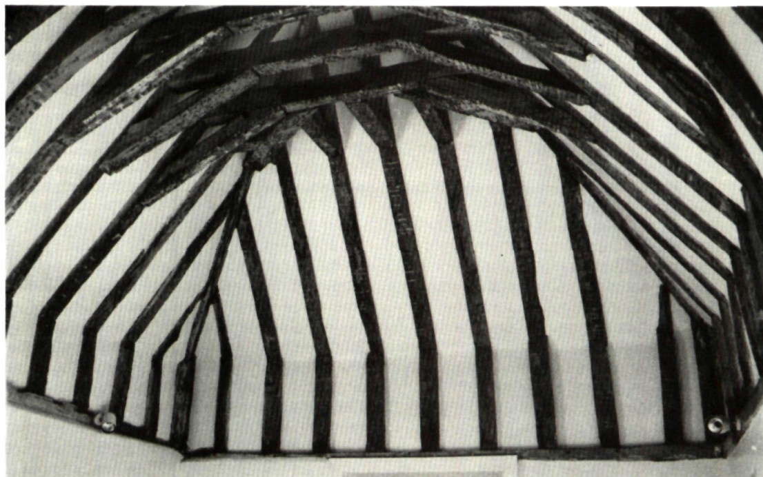
Plate 2. The roof at the west end of the solar range. The timbers here are plain and straight as it was thought unnecessary to create an expensive barrel vault over the probable garderobe (photo: Mr J. Harvey).
