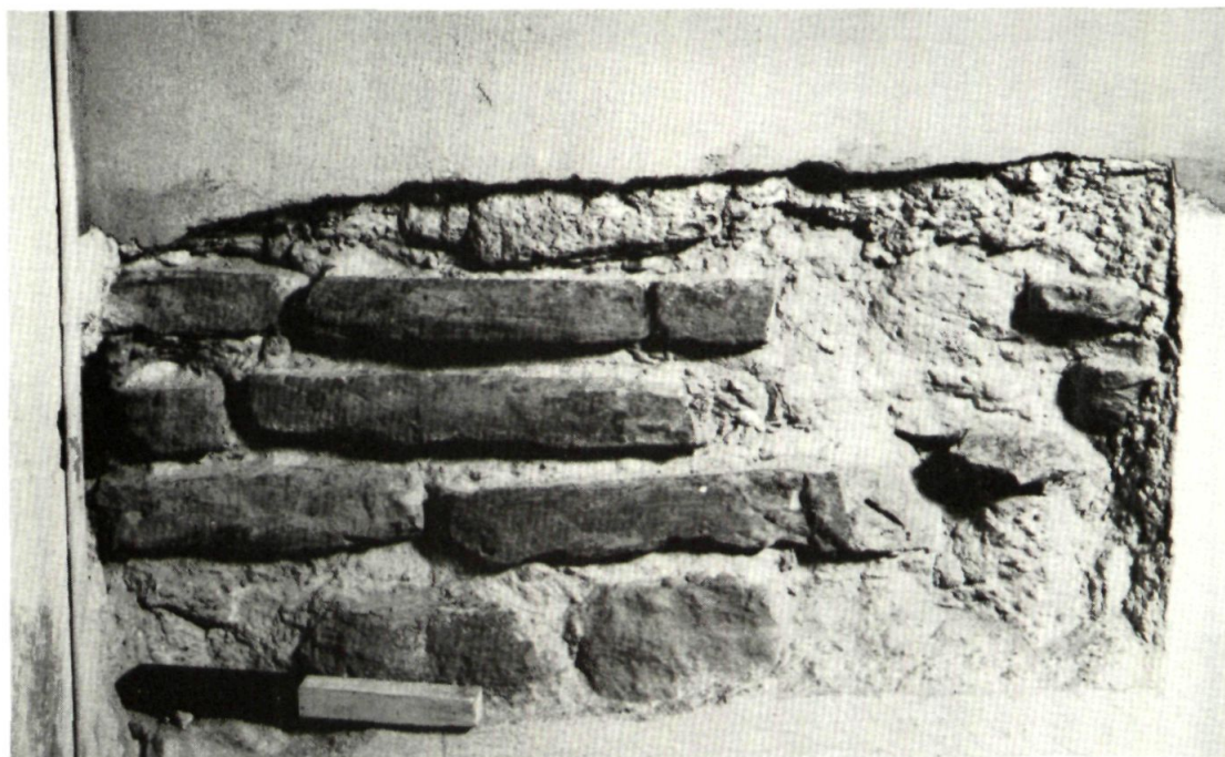
Fig 5. Titchfield church: bonding-course of Roman tiles exposed on the east face of the chancel-arch wall. (Photo: C. Harfield)
