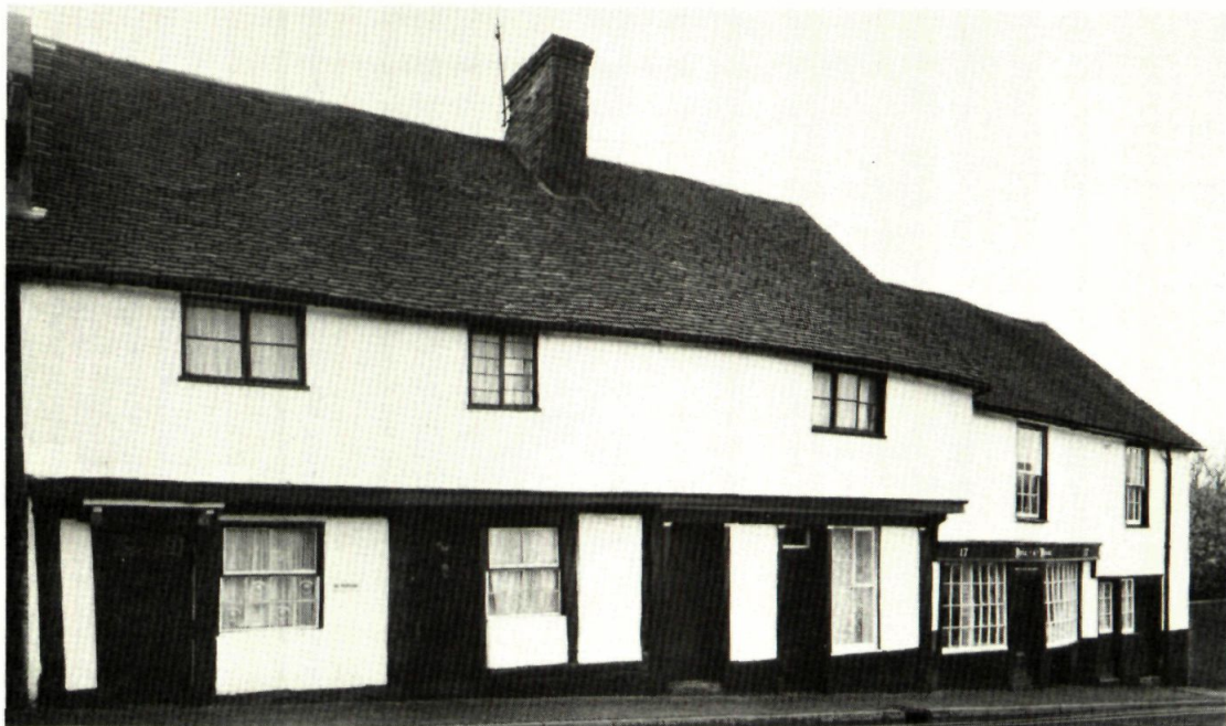
Fig 11. Exterior of 11-13 Chantry Street, Andover (RCHME).
