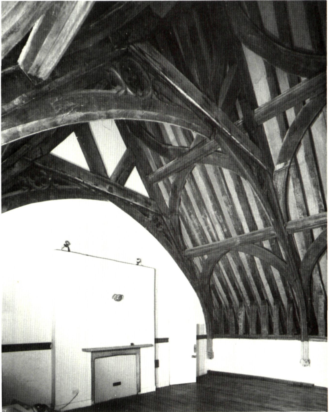
Fig 17. General view of roof of Prior's Hall in second-floor bedroom at south end of hall. Photo: John Crook.
