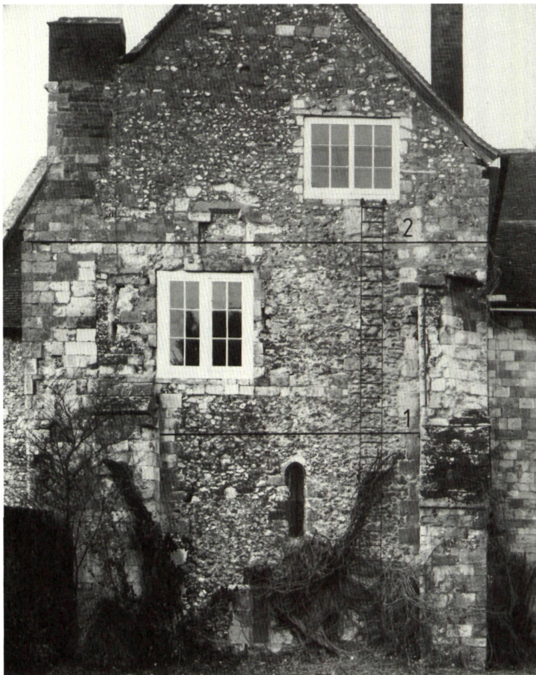
Fig 8. Porch east gable wall. Horizontal lines indicate first and second floor levels. Photo: John Crook.
