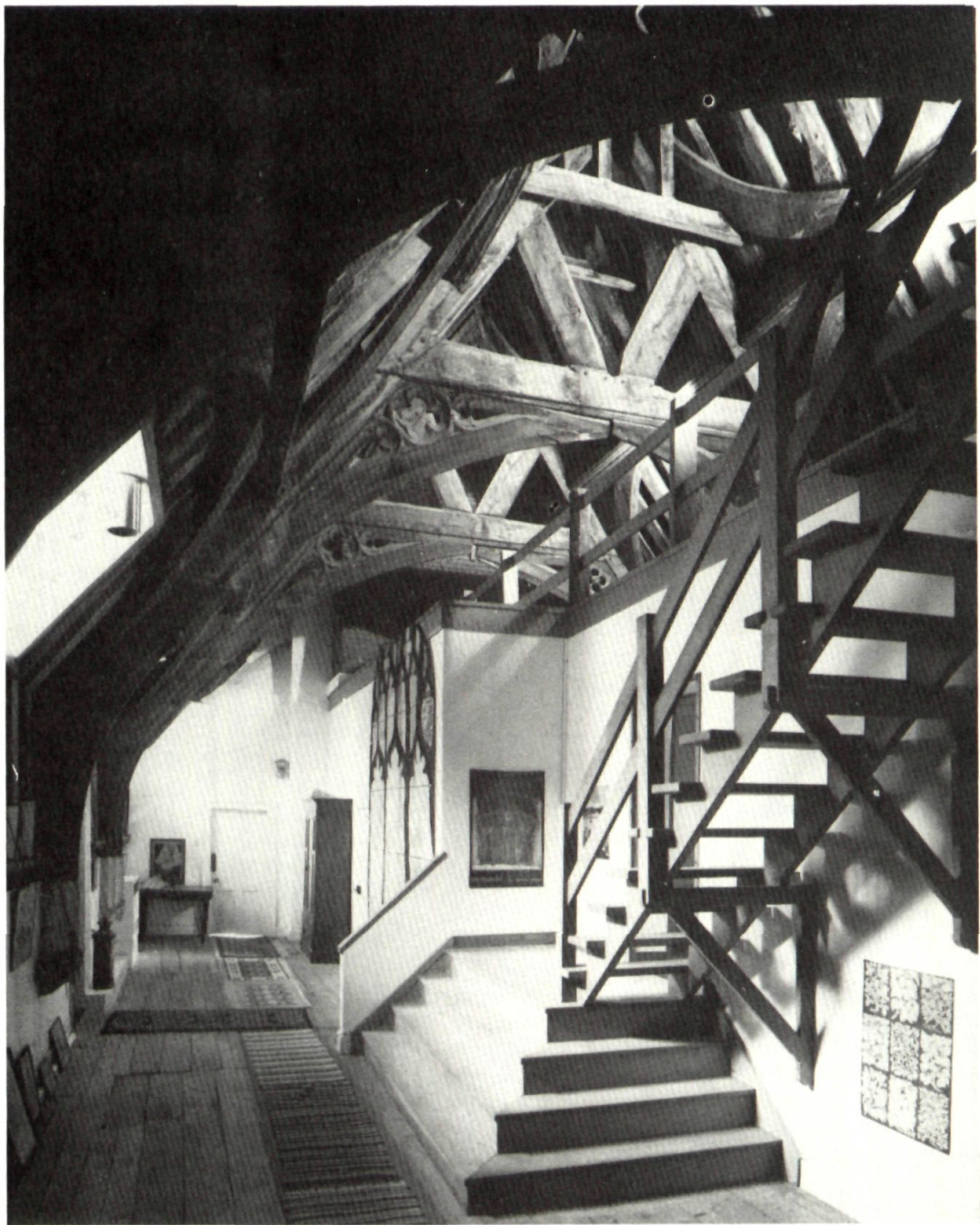
Fig 18. Roof of Prior's Hall from NE corner of hall. Photo: John Crook.
