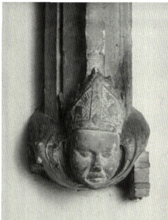
Fig 21. Roof of Prior's Hall. Corbel head of a bishop. Truss IV East. Photo: John Crook.
