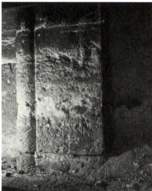
Fig 15. Jamb of first-floor door at NE corner of Prior's Hall, showing rebate (with iron fitting) and external roll-moulded corner. Photo: John Crook.
