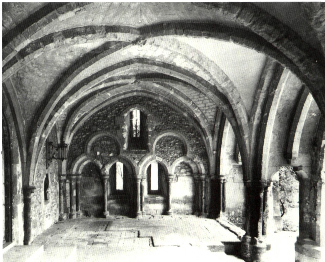
Fig 6. Interior of porch, facing east. Photo: John Crook.
