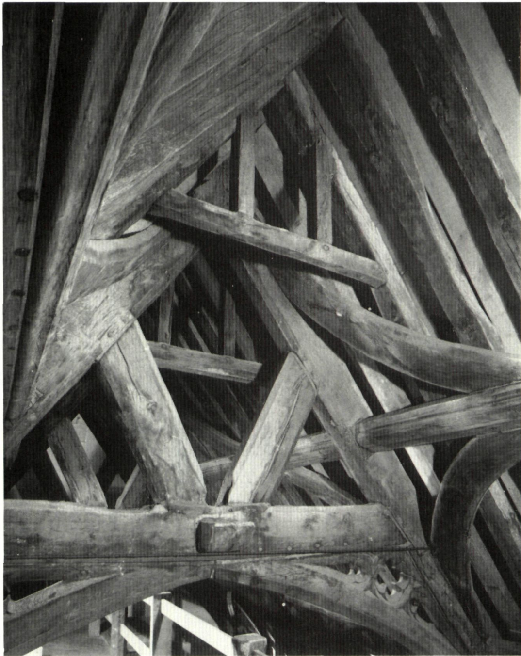
Fig 19. Roof of Prior's Hall. Detail of Truss III and louvre from SW. Photo: John Crook.
