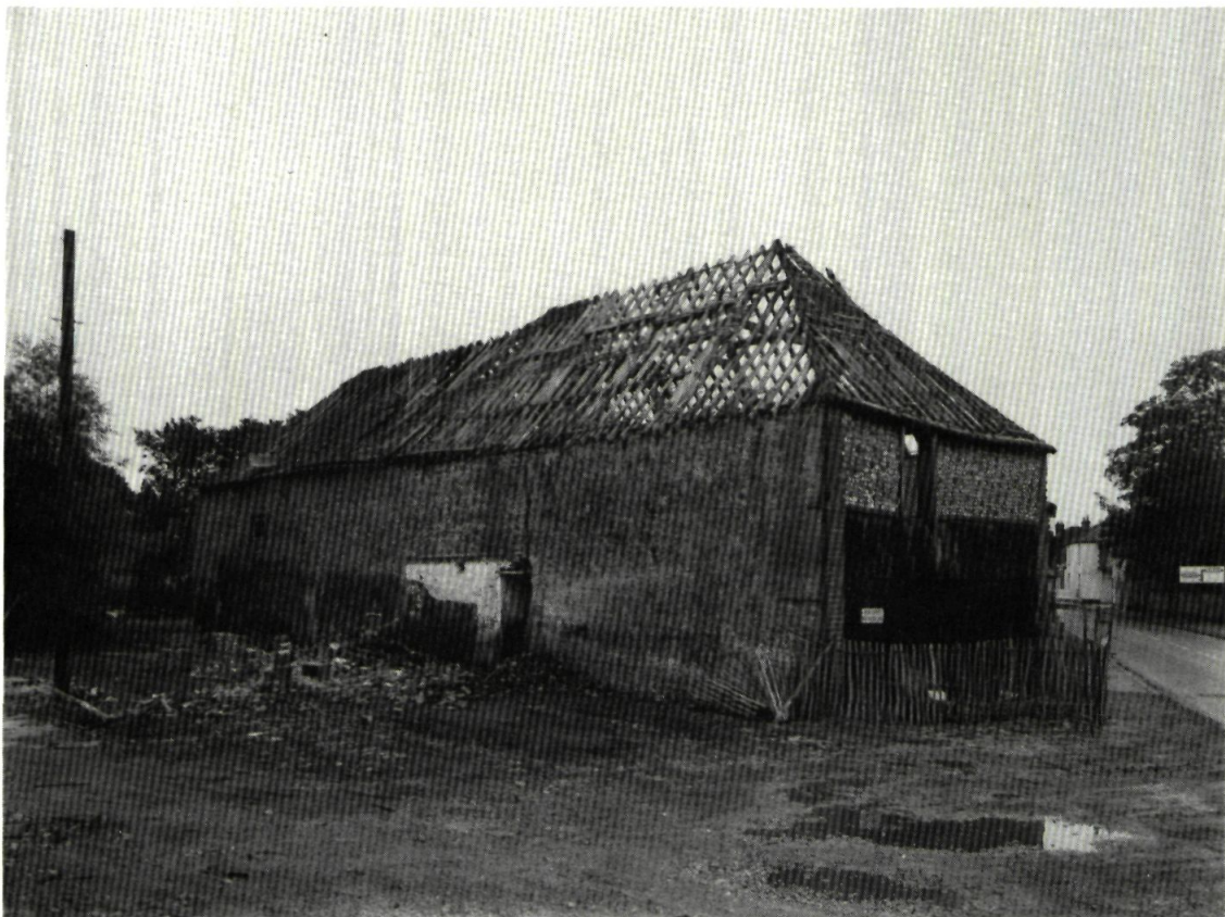
Fig 7. Bishops Waltham: the 'Palace Stables' from the west during demolition, showing the Norman flint wall. Photo: R C H M E.
