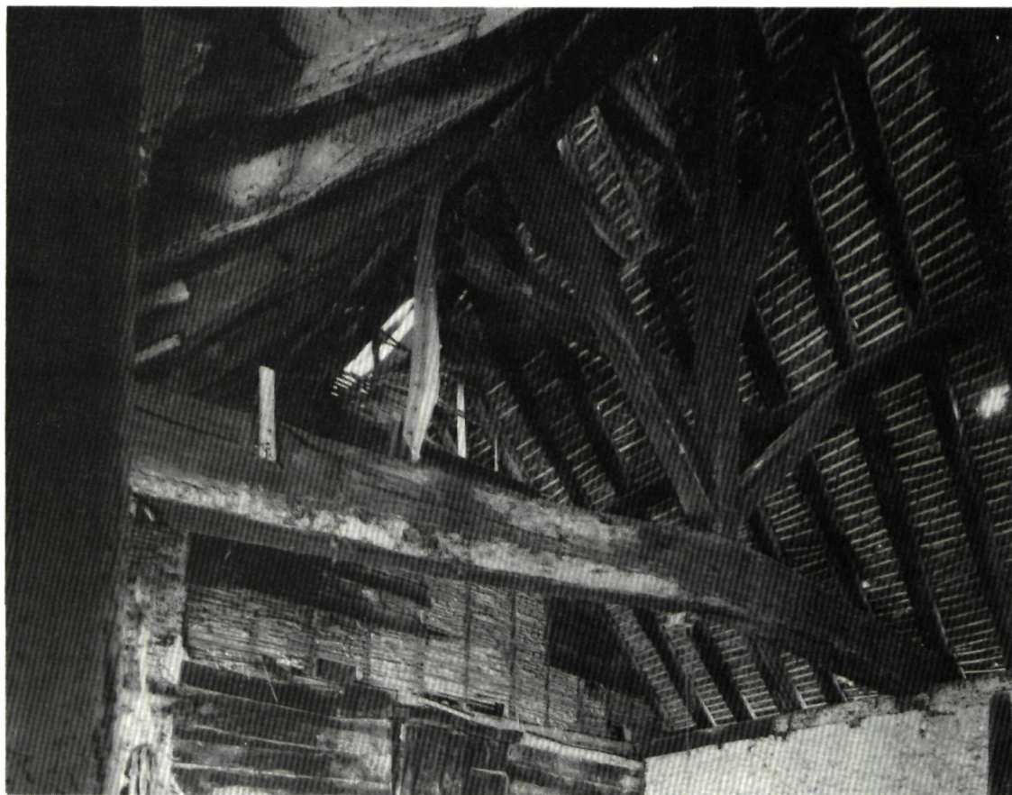
Fig 12. Bishops Waltham: the roof of the 'Palace Stables before demolition. Photo: R C H M E.
