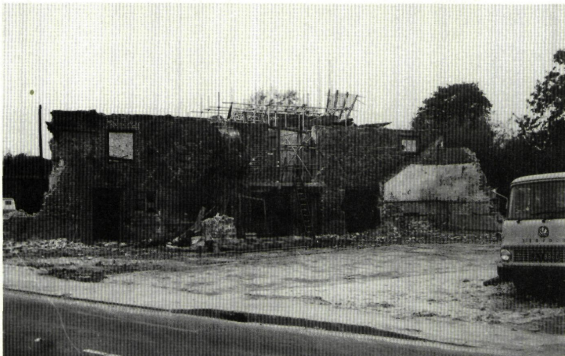
Fig 9. Bishops Waltham: the 'Palace Stables' from the east during demolition, showing the brick wall and buttress of the early sixteenth century. Photo: J. Bosworth.
