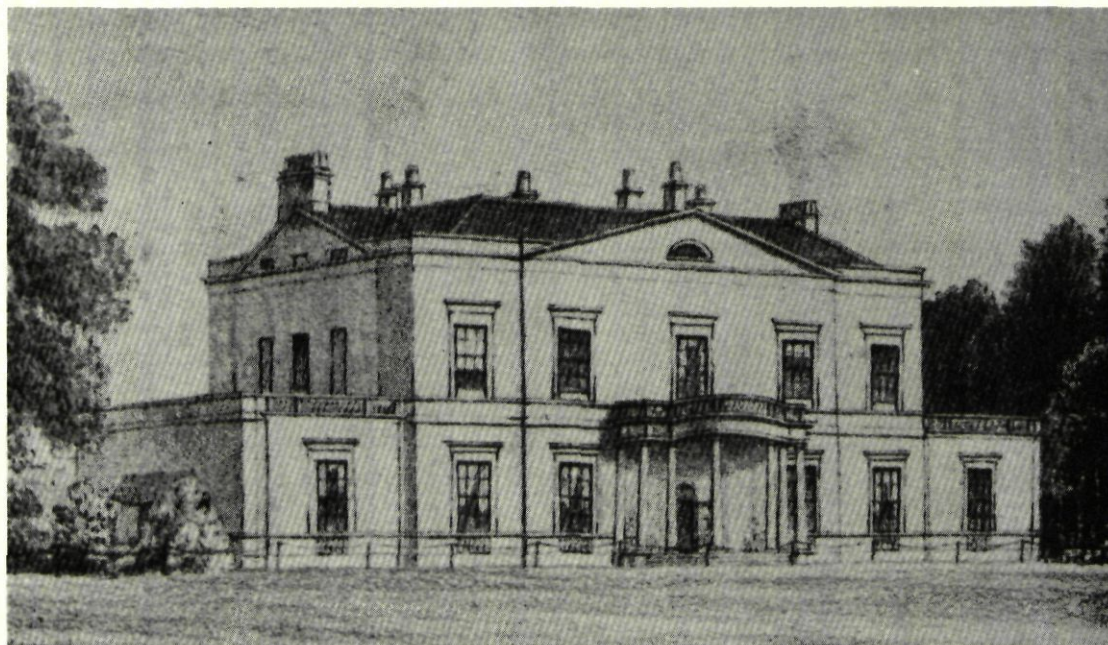
Fig 5. Portswood House c 1840 (SRO SC20/3/2/12).
