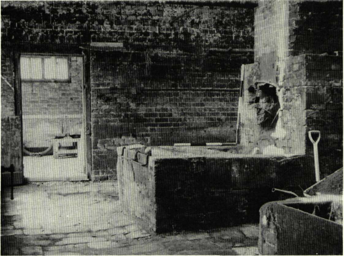
Fig 7. Hook: interior of the smithy in 1975, showing the hearths (Photo: Author).
