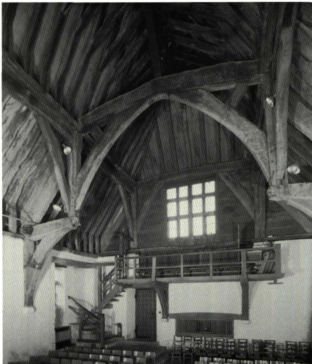
Fig. 1. Pilgrims' Hall, Winchester. Hammer-beam truss V and end truss VII viewed from the south. Photo A F Kersting.
