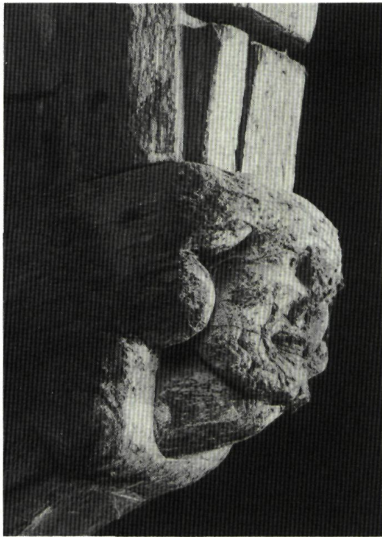
Fig. 10. Pilgrims' Hall, Winchester. Head terminating east hammer beam of truss V.
