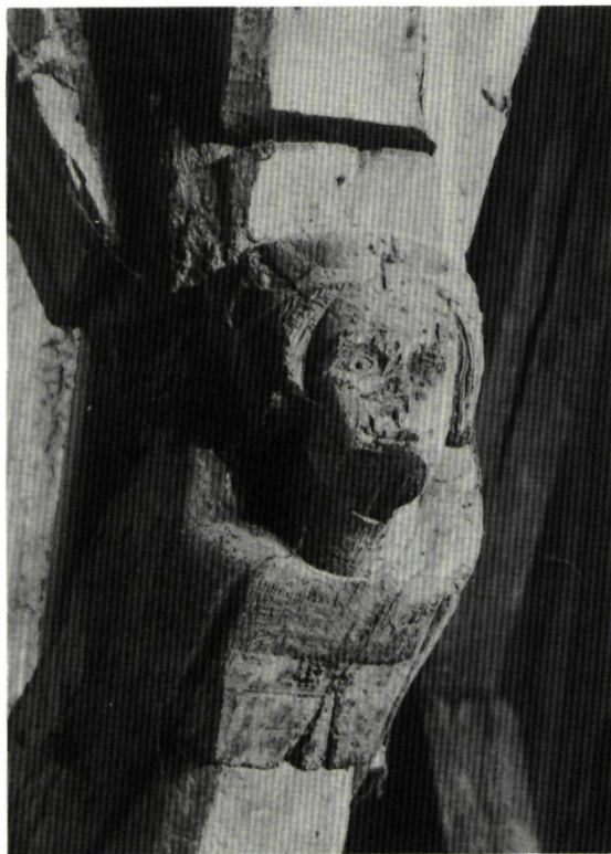
Fig. 9. Pilgrims' Hall, Winchester. Crowned head terminating west hammer beam of truss IV.
