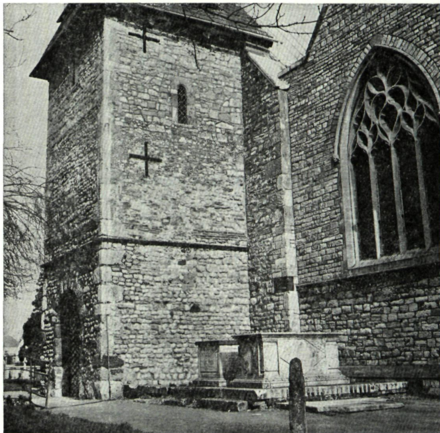
Plate 3. Titchfield Church, tower from south-west. (Photo. A. M. ApSimon.)
