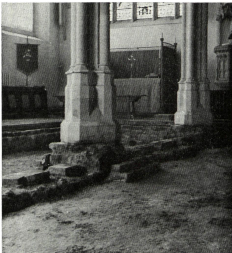
Plate 8. Titchfield Church, photograph taken during repairs in 1955. The photograph is taken from the west end of the nave and shows the east end of the north aisle, with a continuous foundation wall visible beneath the north arcade.
