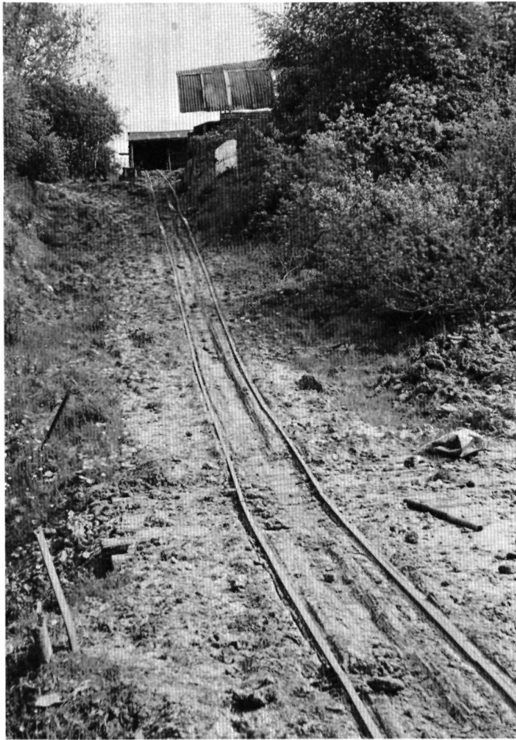
Rope worked incline from pit to pug mill at Selbourne. ( Photo: E. Course. )
