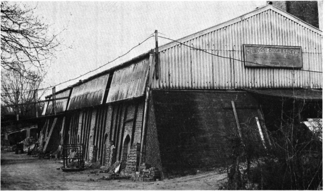
Hoffman kiln at Selbourne. ( Photo: E. Course. )
