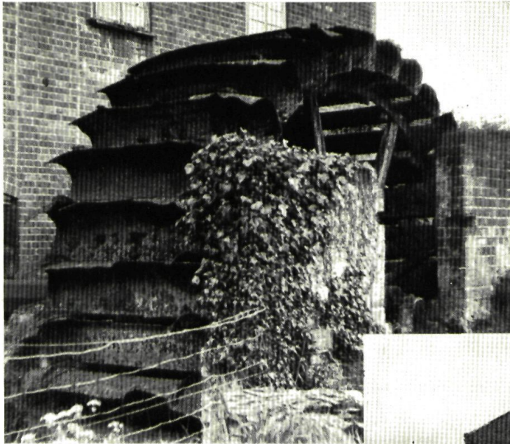
Titchfield Mill, breastshot wheel by Armfield's of Ringwood (page 136).
