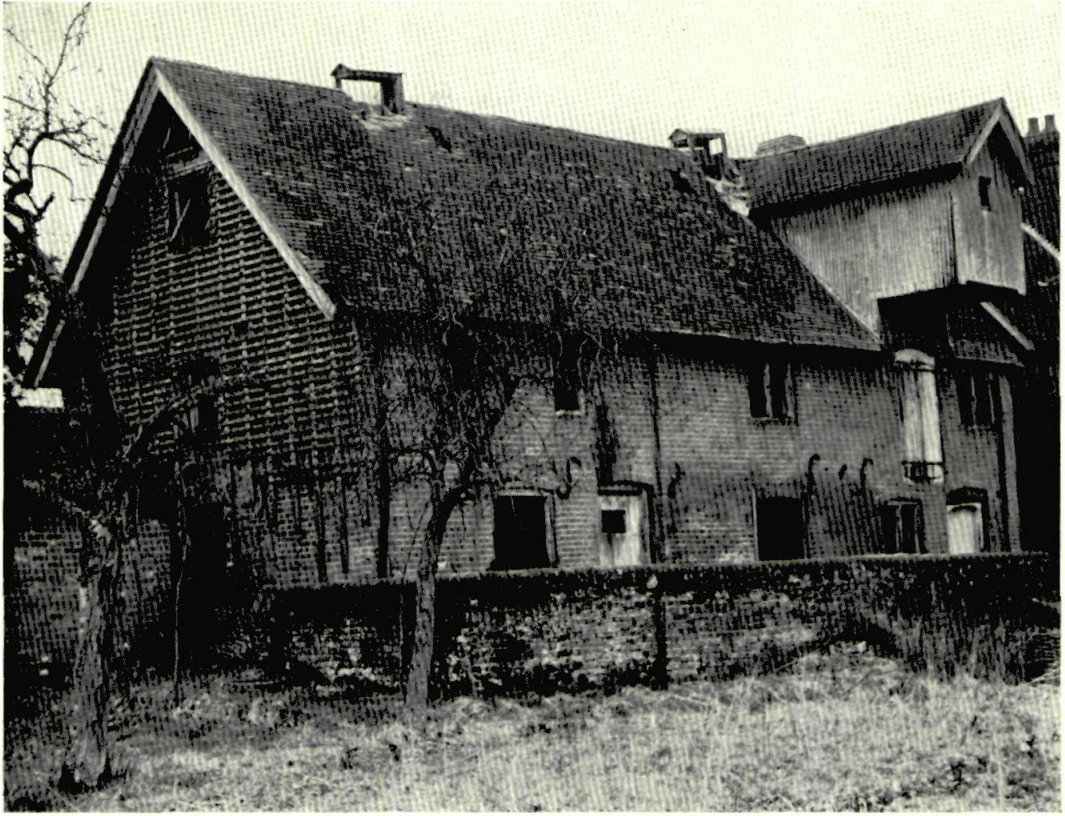
Ford Mill, Lockerley, showing external hoist and ventilating louvres (page 132).
