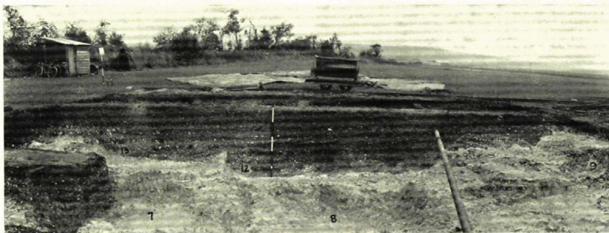
Pl. 9. WEST FACE OF CUTTING III B. (Section Z—Z on Fig. III.)
