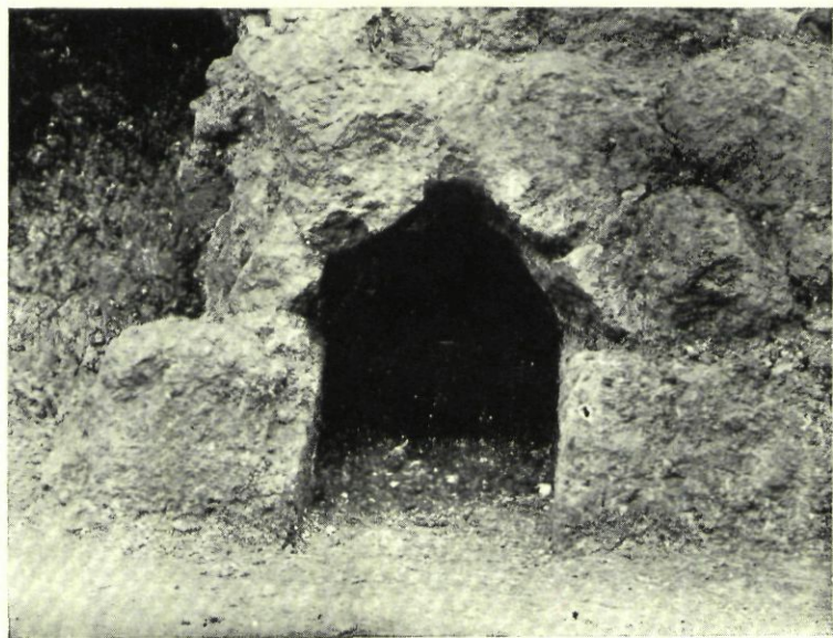
FIG. 12.—SOUTHERN TUNNEL. THE OUTLINE OF THE KEYSTONE IS RATHER OBSCURED BY CLAY BETWEEN THE STONES.
